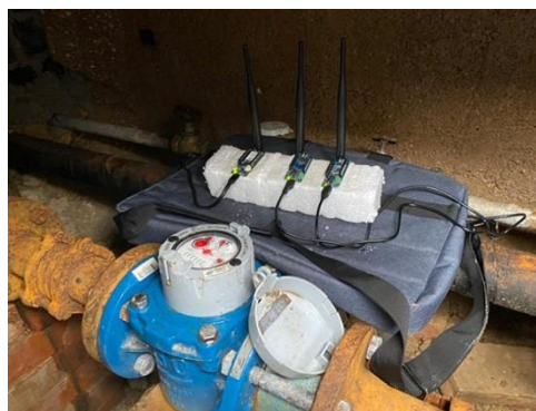
Water meter in Split University
